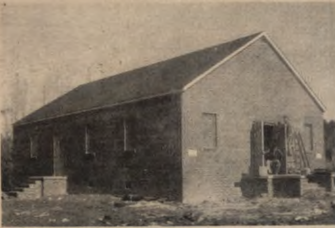
Church nearing completion in Charlotte, North Carolina
