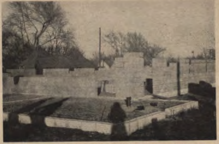
Partially finished church building in El Reno, Oklahoma
