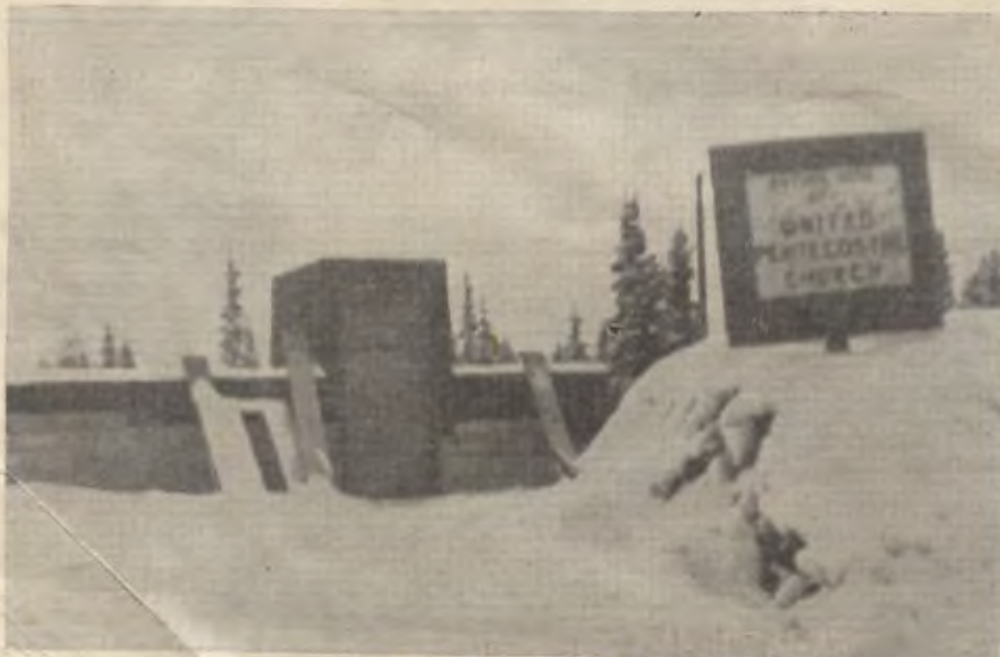
United Pentecostal Church Basement, Fairbanks, Alaska
